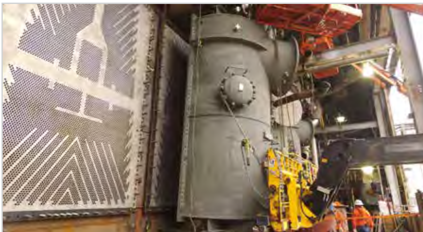
Steam Surface Condenser Modular Changeout
